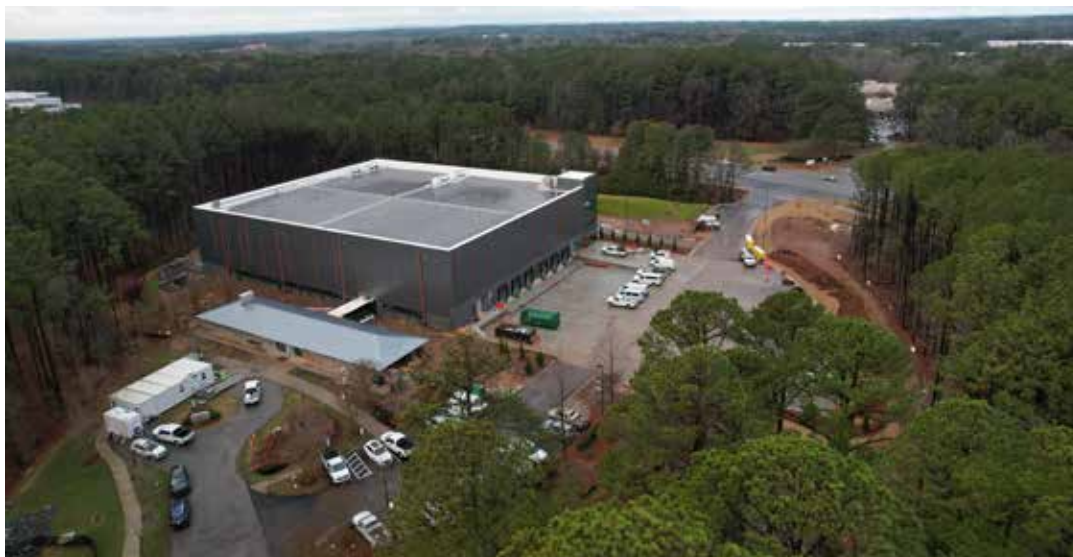
Figure 6: Aerial progress photo.
