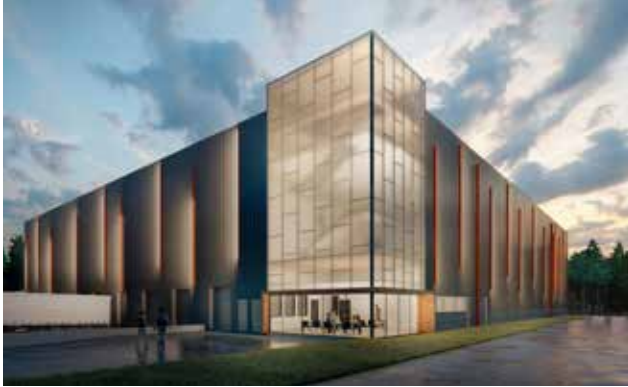
Figure 2: Project rendering of design expected to meet the desired net zero energy goals.
